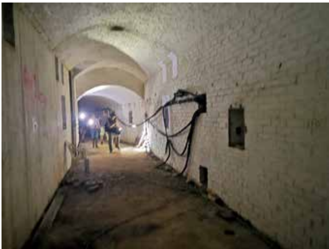
Inside the casemates are shell stores and powder magazines with connections to the emplacements via shell lifts and access ways.
