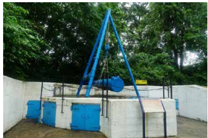
6 in QF emplacement with a replica 6 in barrel being lifted at Fort Siloso.
