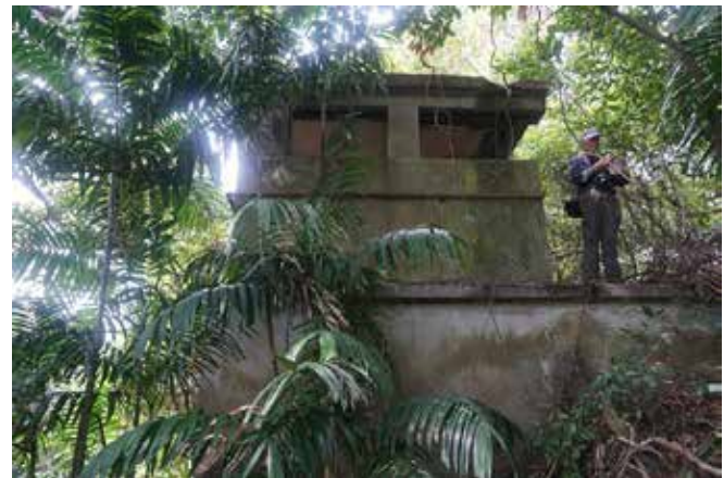
Secondary battery observation post at Fort Connaught.
