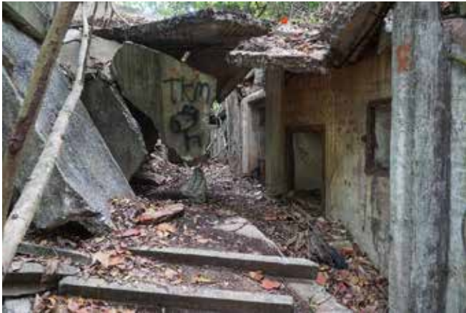
Serapong Spur 9.2 in emplacement with the collapsed 6 in gun overhead protection.
