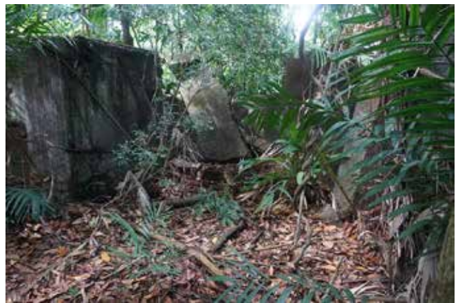
Damage to Fort Connaught's Gun Emplacement #3 caused by spiking or the removal the guns when they were scrapped.
