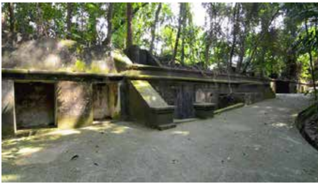
The 6-pounder QF emplacement using the older 7 in RML structure at Fort Passeir Panjang.
